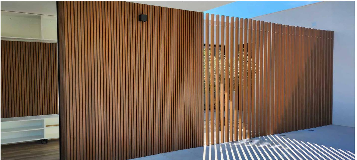
WEO Brise Soleil are architectural elements designed to regulate the flow of light. Their adjustable gap affects the direct intensity of solar radiation. They are suitable for facade cladding or various decorative applications. They also add an very good looking but do not contribute to the structural performance of buildings.
